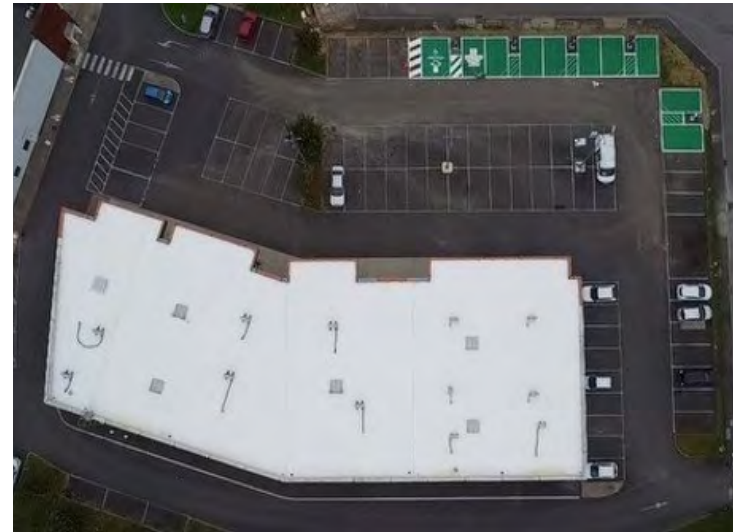
Aerial view of the roof
