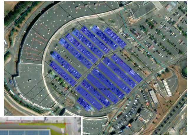
Poitiers: 17,000 sqm of shade structures in car parks, with a total capacity of 3.4 MW
