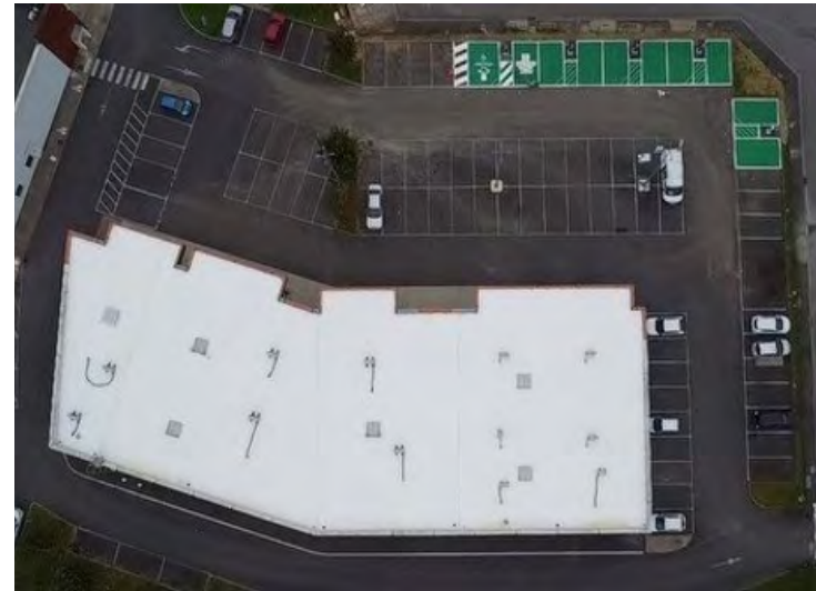
Aerial view of the roof
